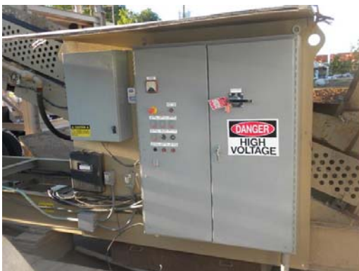
Pugmill Control Panel and Pugmill Mixing Box
